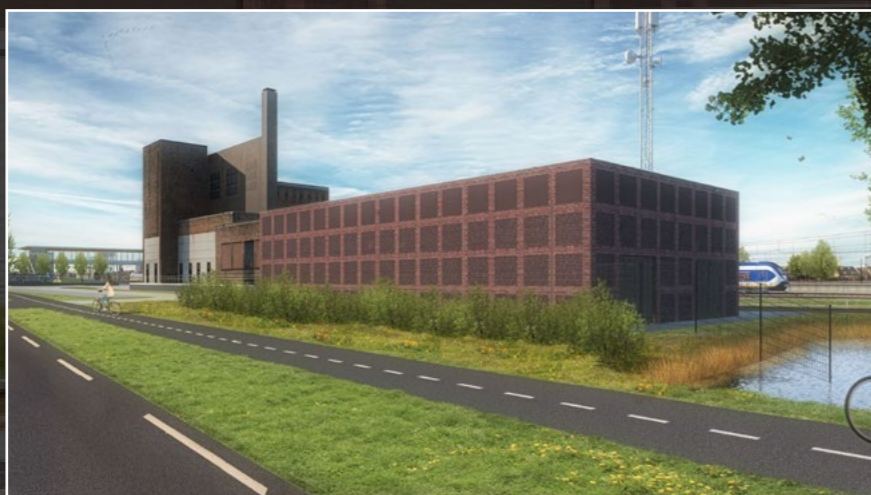
Onderstation, Studio SK
